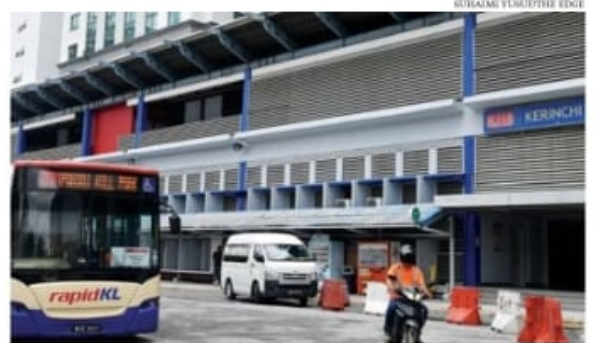
The Kerinchi LRT station is one of the transport hubs in the area
