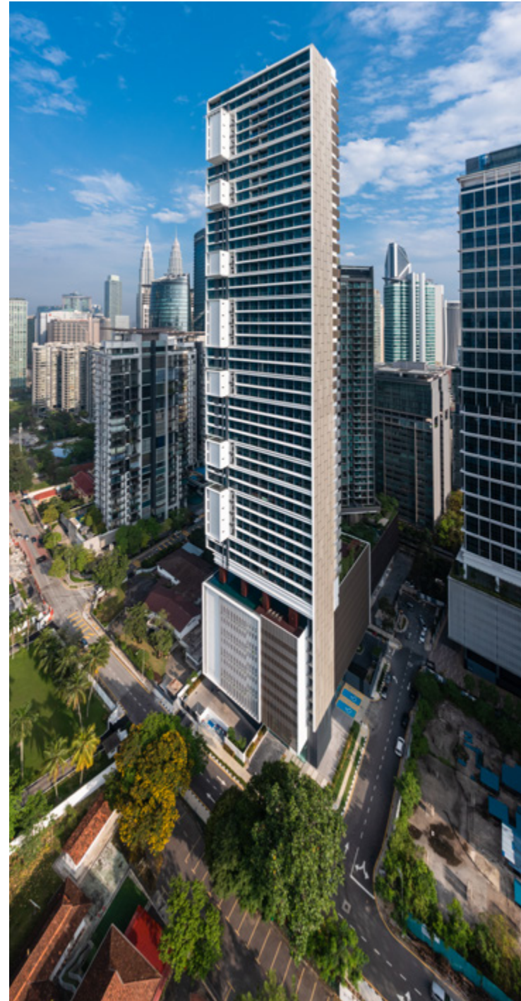
The overall building orientation is set to address the predominant site condition. Avoiding northward views due to close proximity with neighbouring high-rises, the Main Façade is orientated towards Persiaran Stonor (south elevation).
