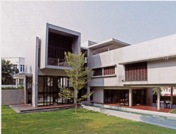
'House Without Finishes' Working within a limited budget, finishes were carefully selected to express their true characteristic and to create a timeless effect. Some of the design strategies used include polished concrete floor and colour skim coat for all walls. There are no glass windows in the bedroom. Instead, two layers of timber louvers are used.
