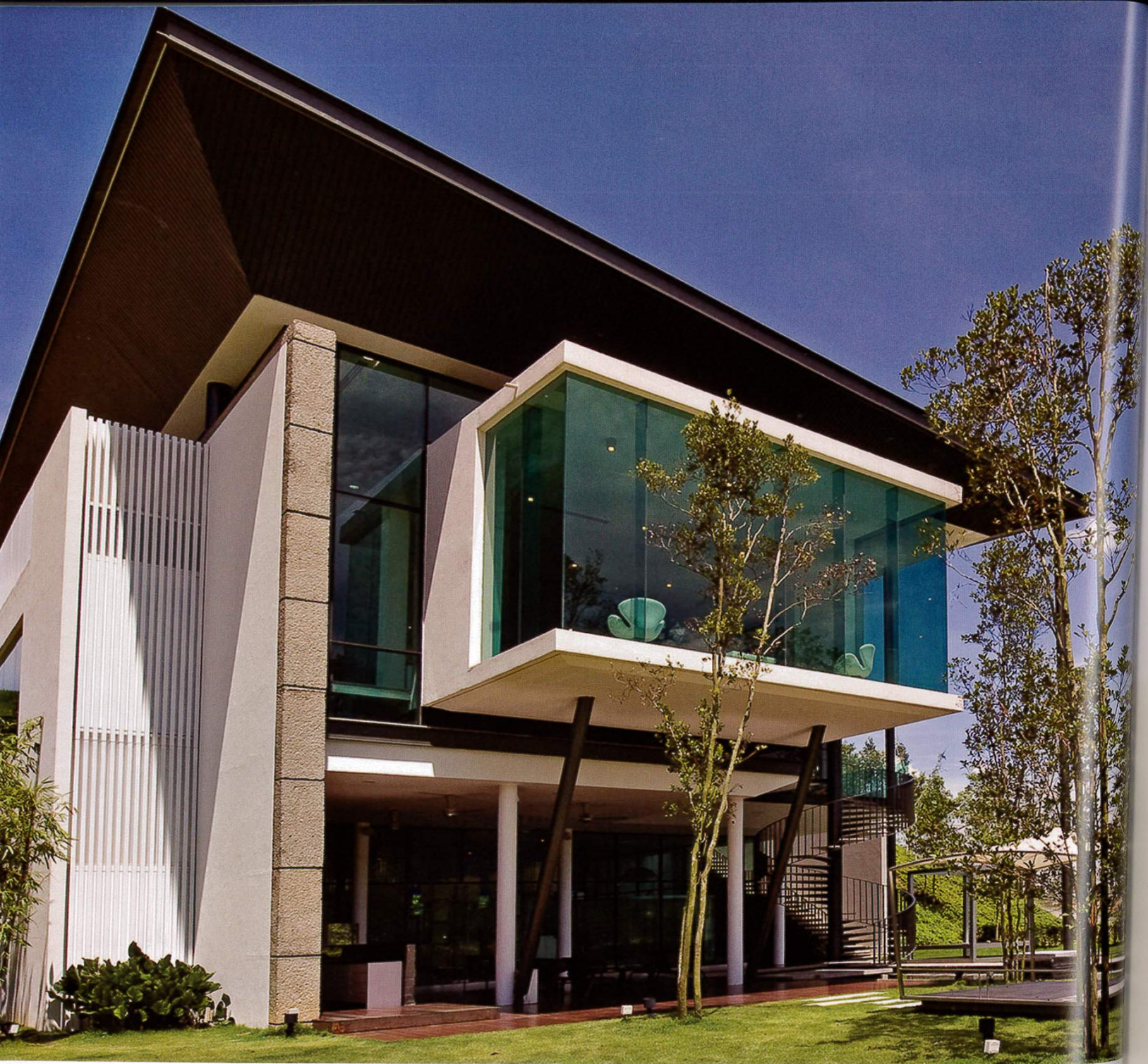
'Nadaya Melawati Sales Gallery' The architectural spatial composition and circulation as well as the façade are designed around this sales lounge specifically to exhibit and present magnificent views to the potential purchaser.
